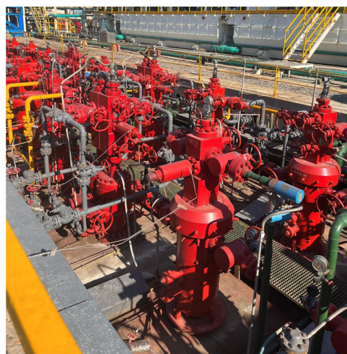
(a) Schematic of the ESP system (b) Surface wellhead equipment and associated manifolds
