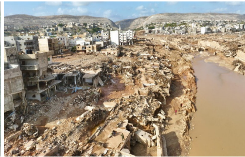
(b) Derna Dam Collapse, Libya
