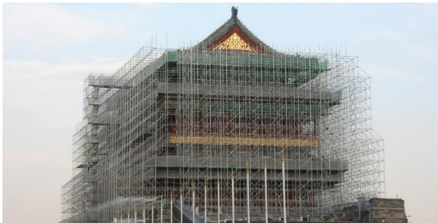
Fig 1. Real scene of Zhengyangmen Gate Tower restoration project (image source: internet)
